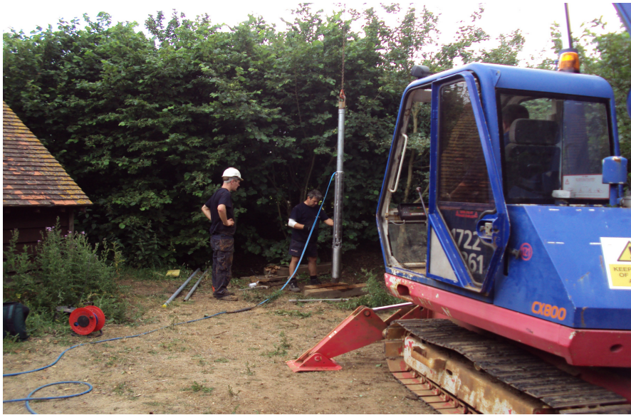
Installing new borehole pump
